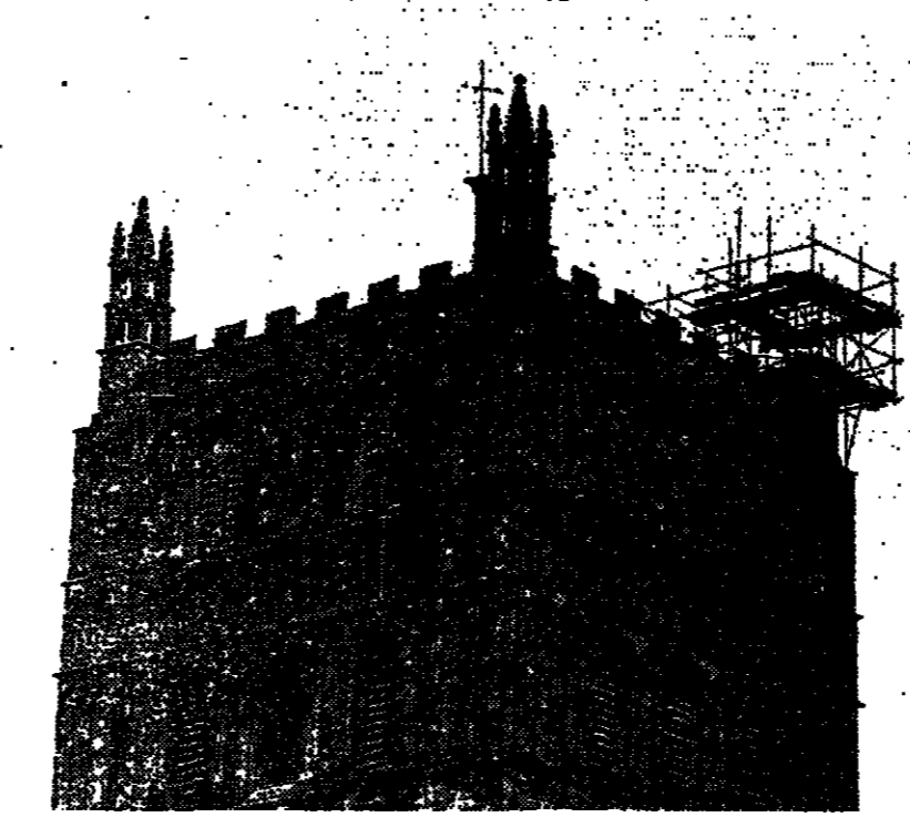
Four tons of stone being lifted by RAF helicopter to the top of the great Norman tower of Tewkesbury Abbey to replace the south-west pinnacle, which had to be taken down after gale damage. The tower, completed about 1145, is believed to be the largest Norman tower extant.
